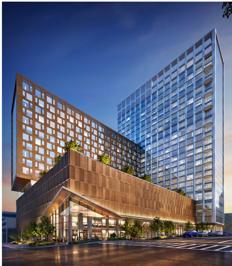
Current LRC Project: 25 North Lexington Ave., White Plains
